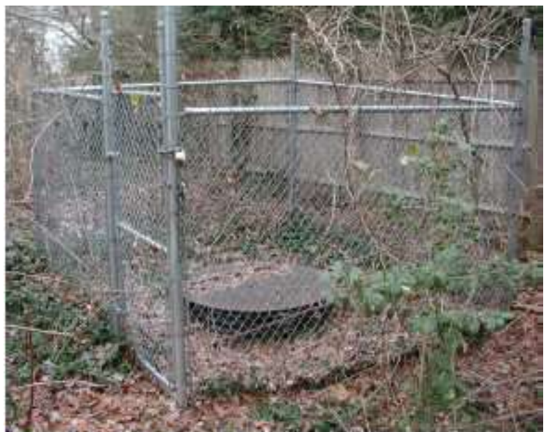
John's Pond Outlet Control Structure Marine Fisheries photo
