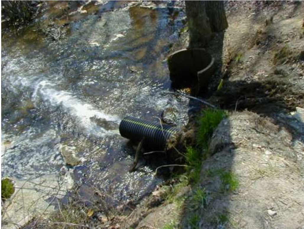
Pond outlet at River Rd.
